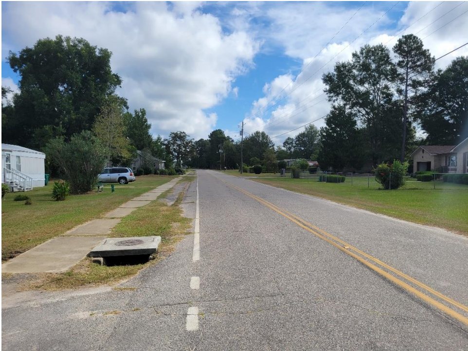
Figure 8. Typical Drainage Inlet Along Sumter Street
