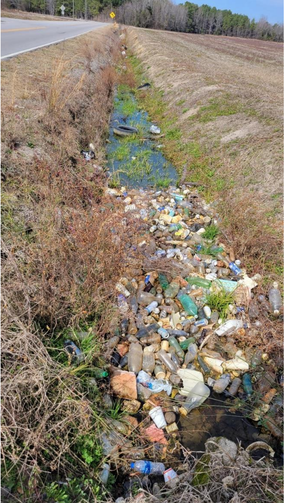
Figure 20. Drainage Channel Along Avenue A
