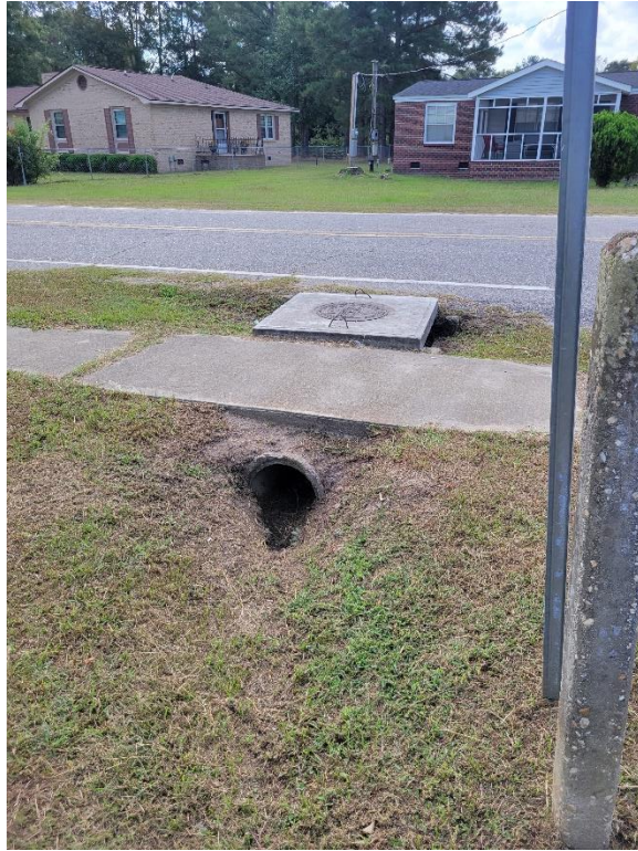
Figure 10. Typical Drainage Inlet Along Sumter Street
