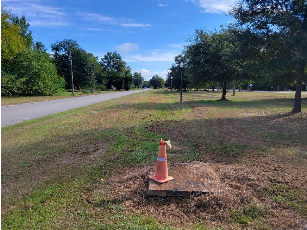
Figure 6. Typical Drainage Inlet along Main Street
