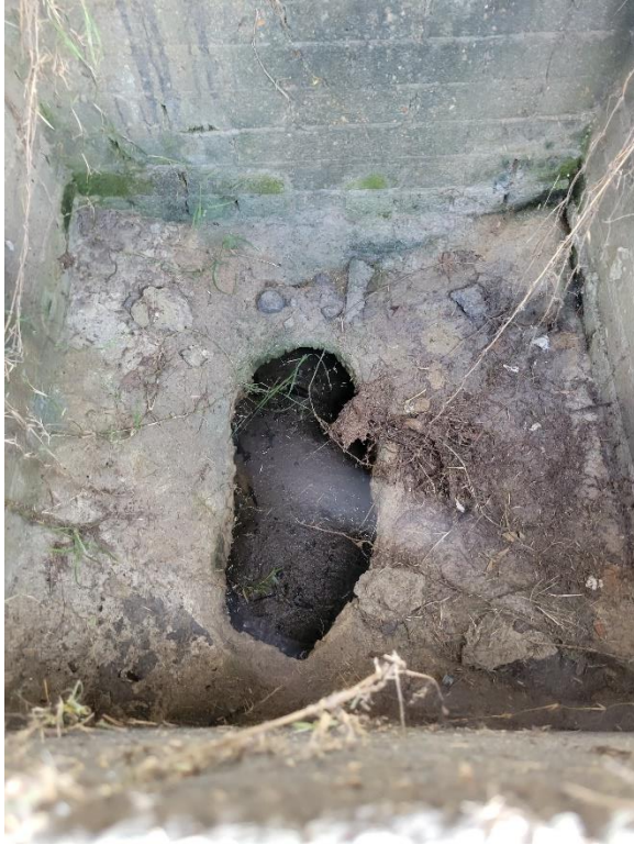
Figure 9. Typical Drainage Inlet Along Sumter Street
