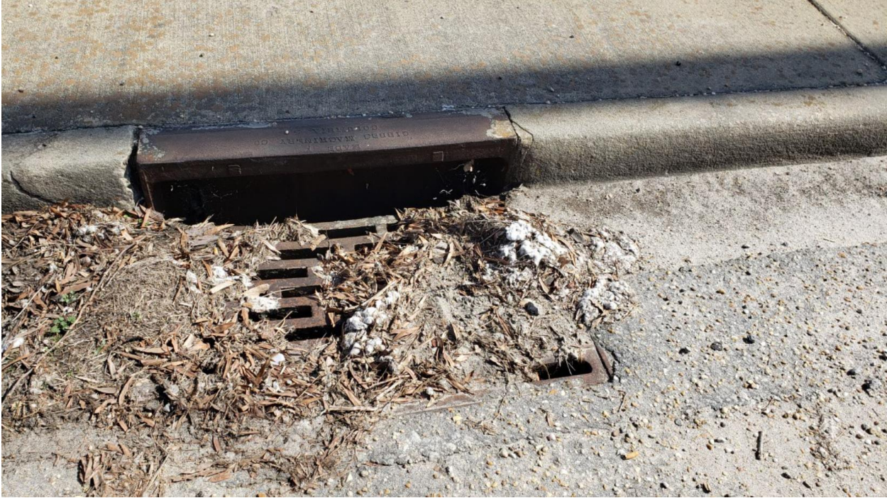
Figure 16. Typical Drainage Inlet along Lafayette Street
