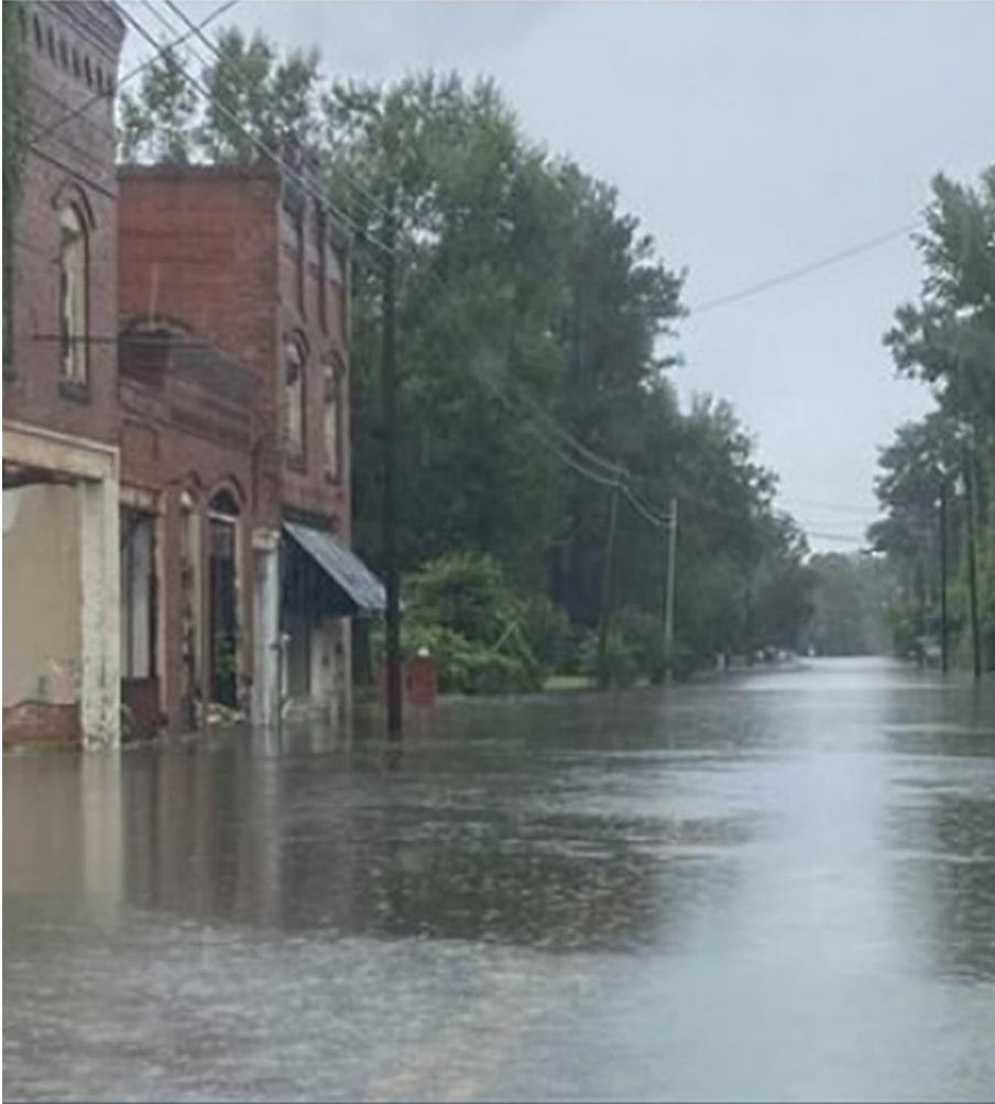
Figure 2: Photo of flooding from Hurricane Sally in the Town of Mayesville, 2020
