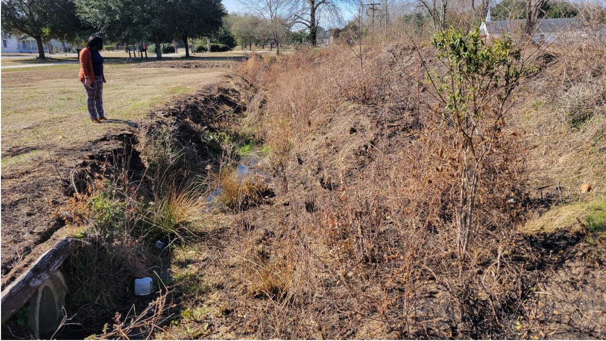
Figure 18. Drainage Channel Along Walking Trail
