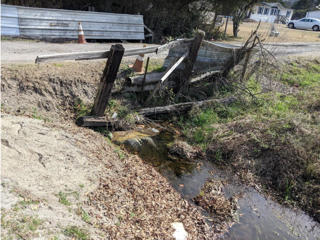
Figure 21. Culvert under private drive at the end of Avenue B
