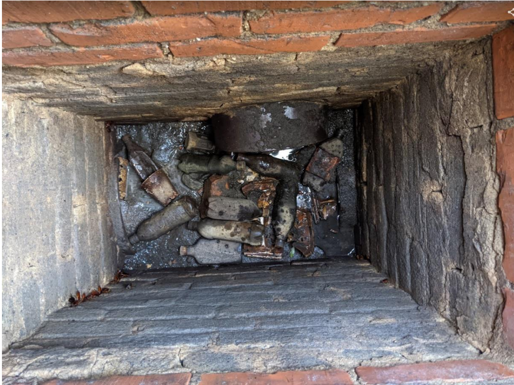
Figure 5. Catch basin along Main Street
