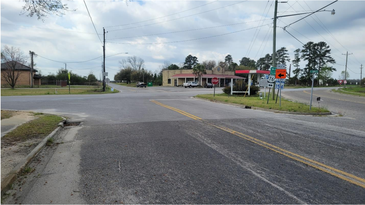
Figure 24. Lafayette Street at US 76
