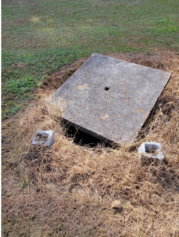
Figure 7. Drainage Inlet along Main Street
