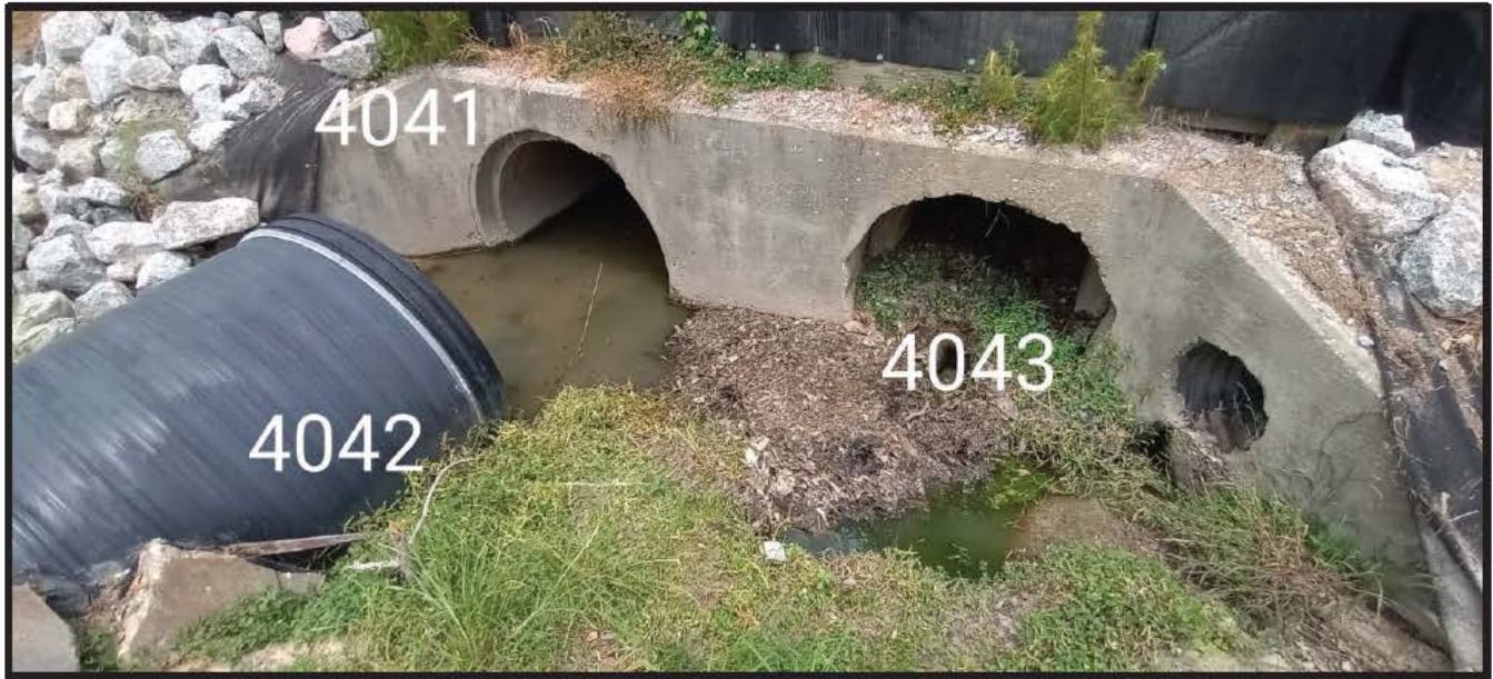
Figure F2: Downstream end of the closed drainage system running parallel to the Blanton Court Mullins Housing Authority Area
