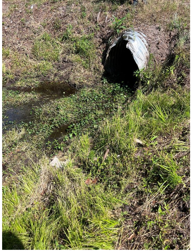
Downstream face of existing 48in CMP
