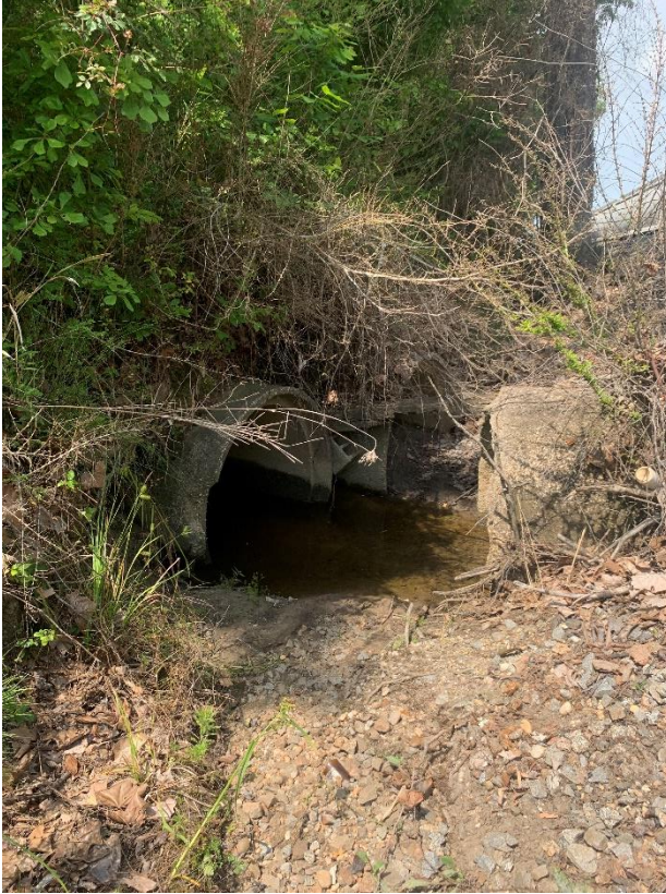
Downstream end of double 48in RCP
