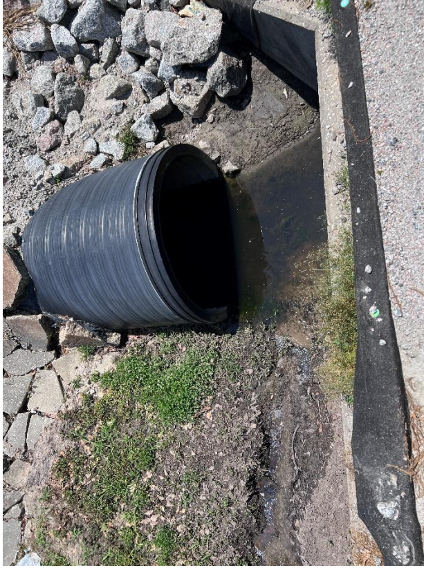
Upstream face of existing 48in HDPE pipe
