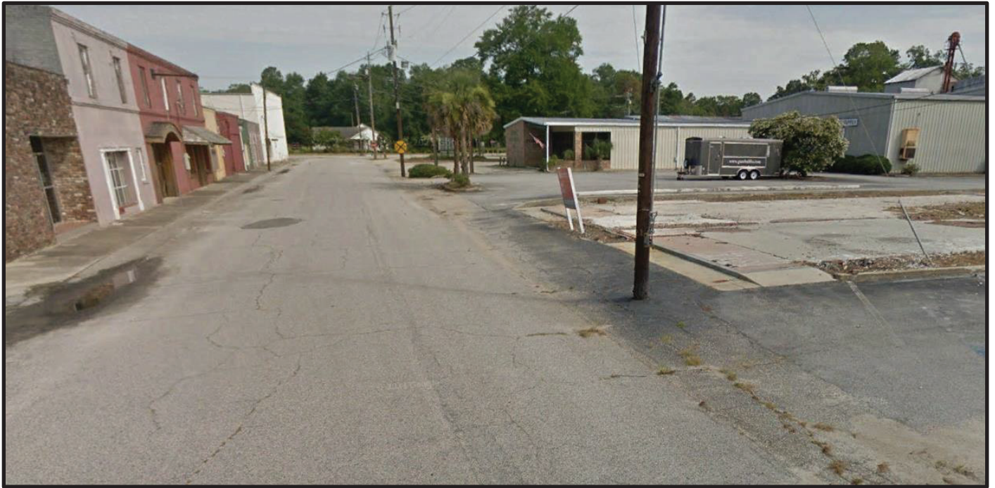
Figure O5: Expansive impervious areas along S. Nichols Street. Note sedimentation and standing water along valley gutters.
