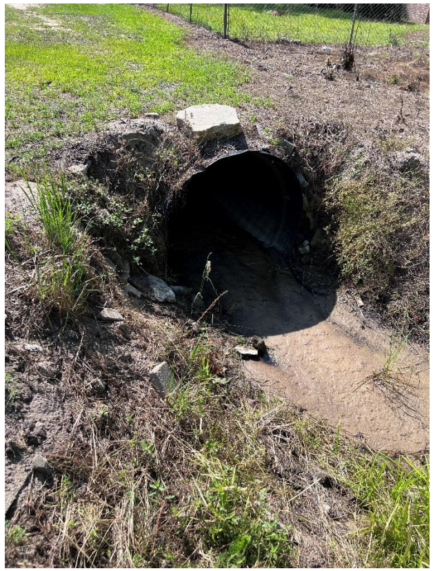
Upstream face of existing 48in HDPE pipe
