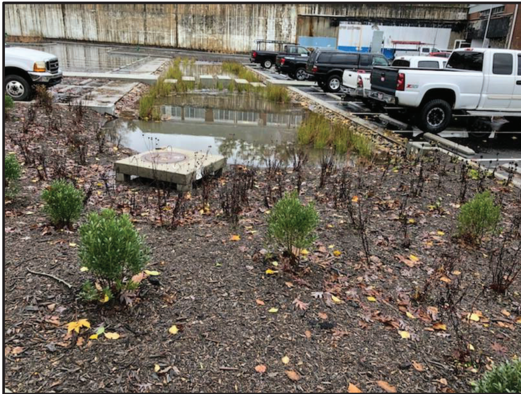
Figure O7: Retrofit bioretention cell designed by MBI shortly after a rain event.
