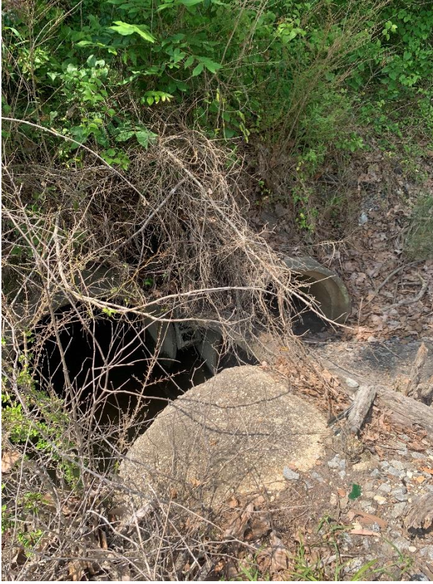
Downstream end of double 48in RCP
