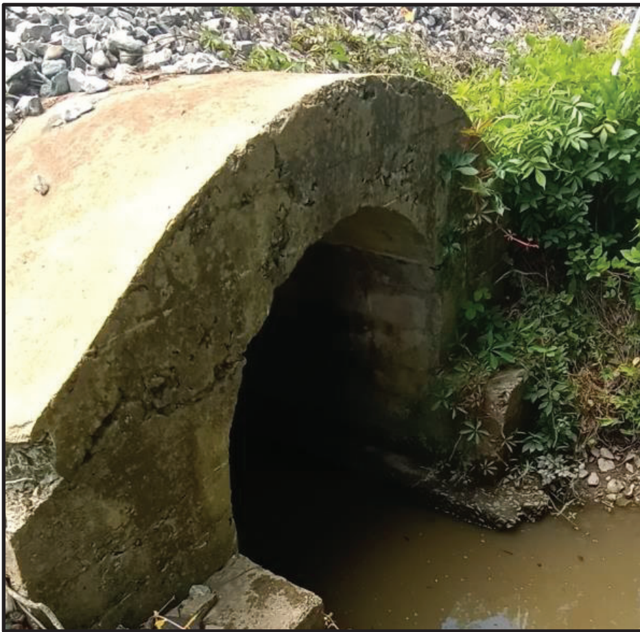
Figure A3: Existing single 48" x 60" cast in place arch pipe under the railroad
