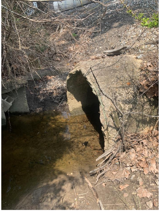
Downstream end of single 48in RCP under railroad
