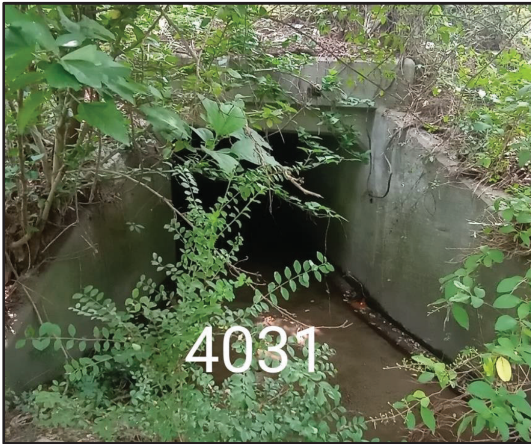
Figure H2: Upstream face of existing box culvert under East McIntyre Street
