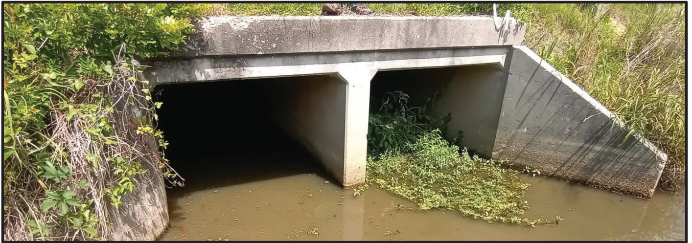
Figure A2: Existing double 6'(W) x 5'(H) box culvert under Highway 301
