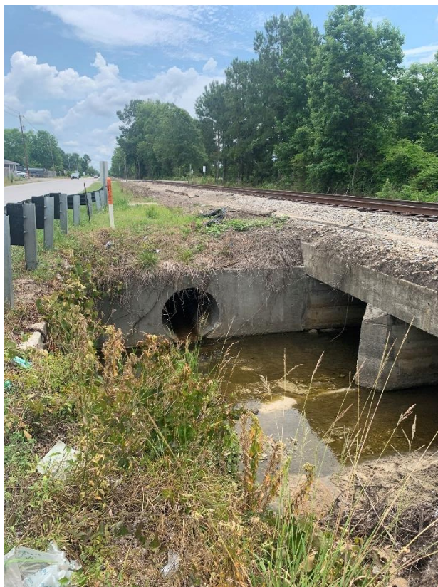
Circular culvert draining to stream
