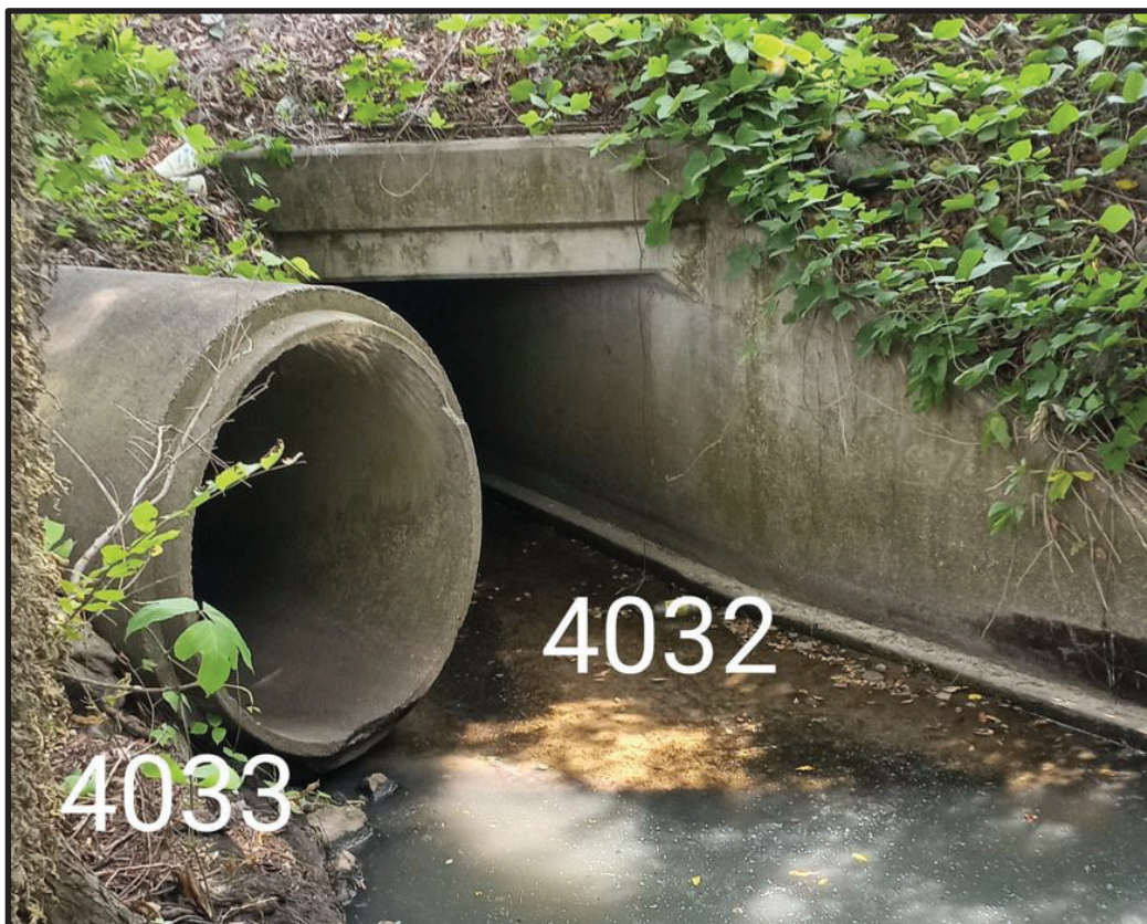
Figure H3: Downstream face of existing box culvert and 48" RCP under East McIntyre Street
