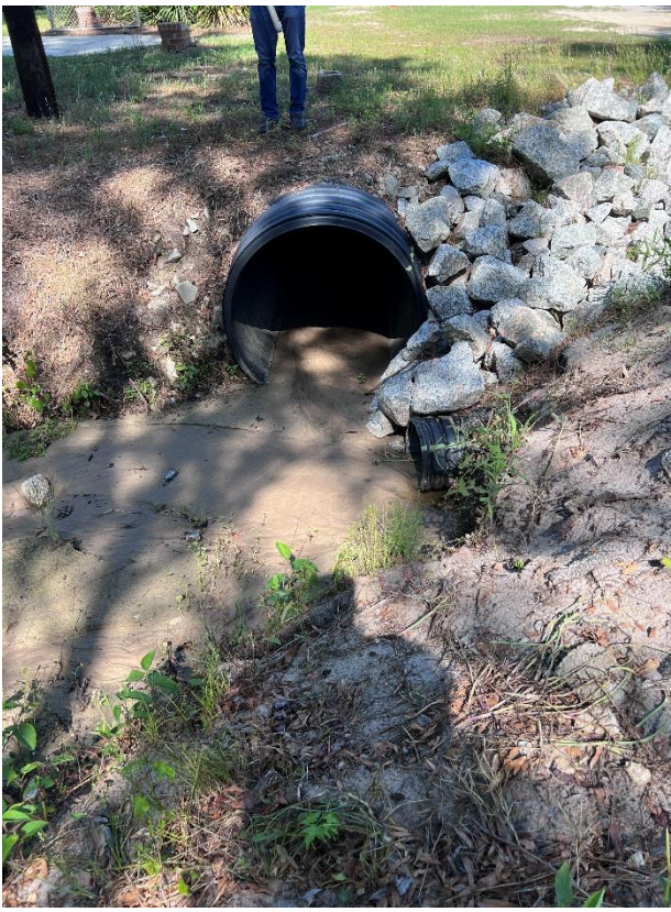
Upstream face of existing 48in HDPE pipe
