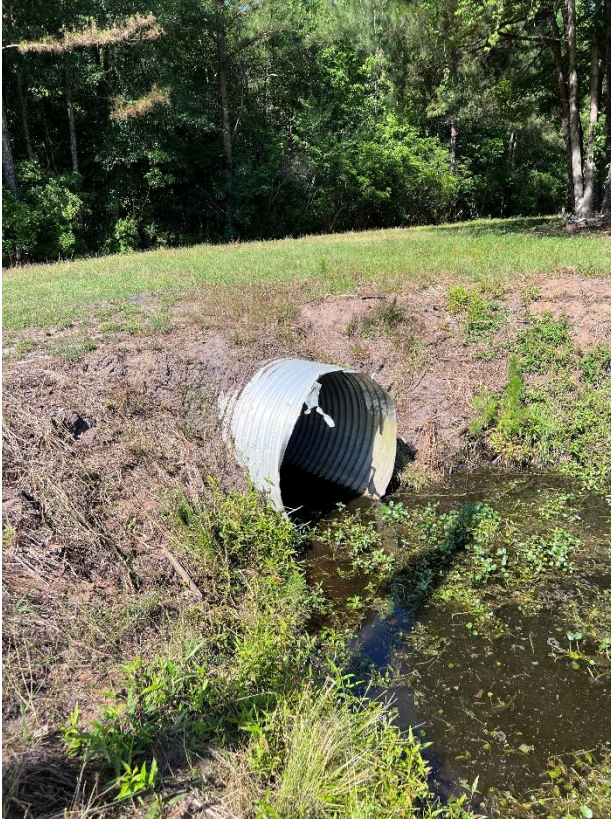
Upstream face of existing 48in CMP
