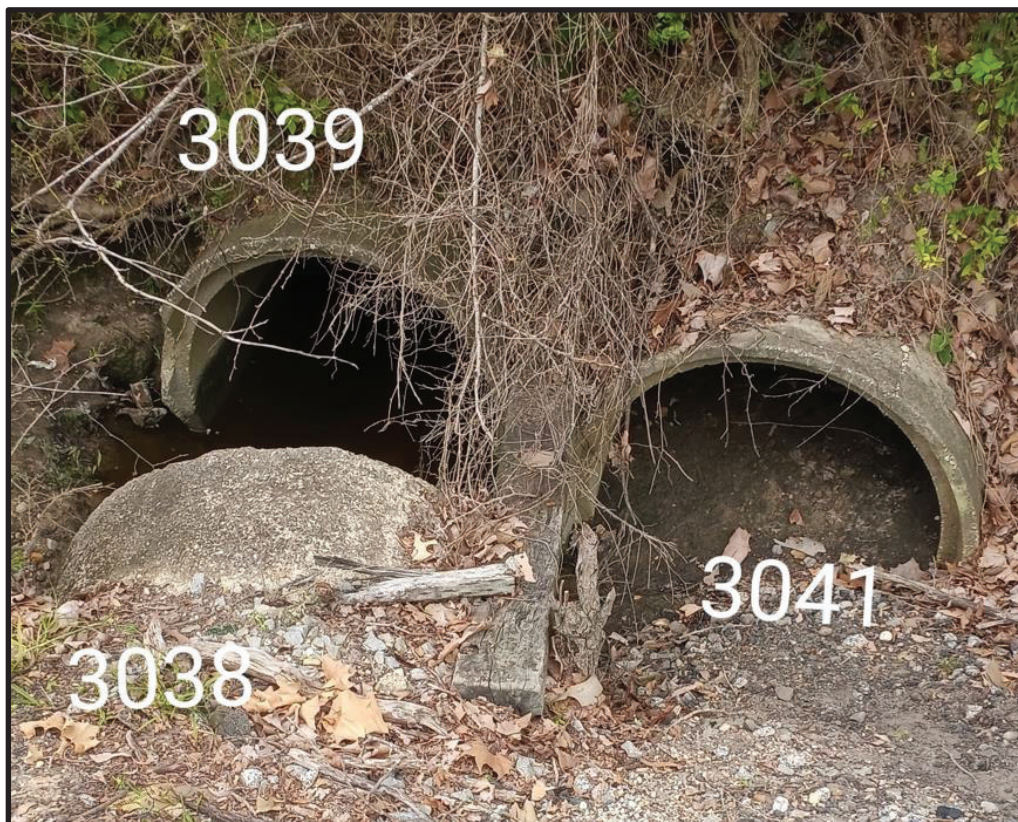
Figure G3: 48" concrete pipe from under the railroad draining to double 48" pipes immediately downstream
