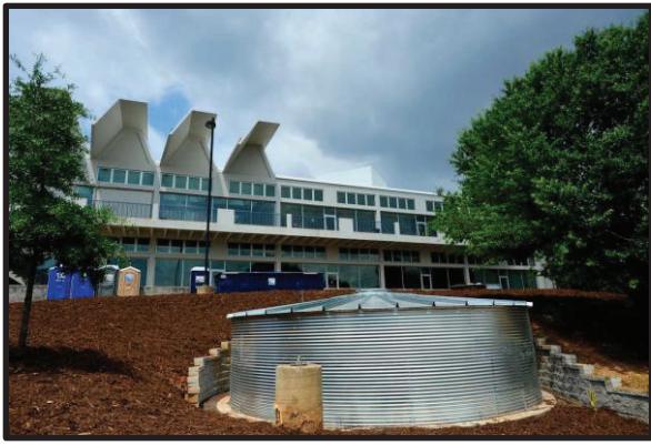
Figures O3A & O3B: Above ground cisterns on a sloped and a flat site.
