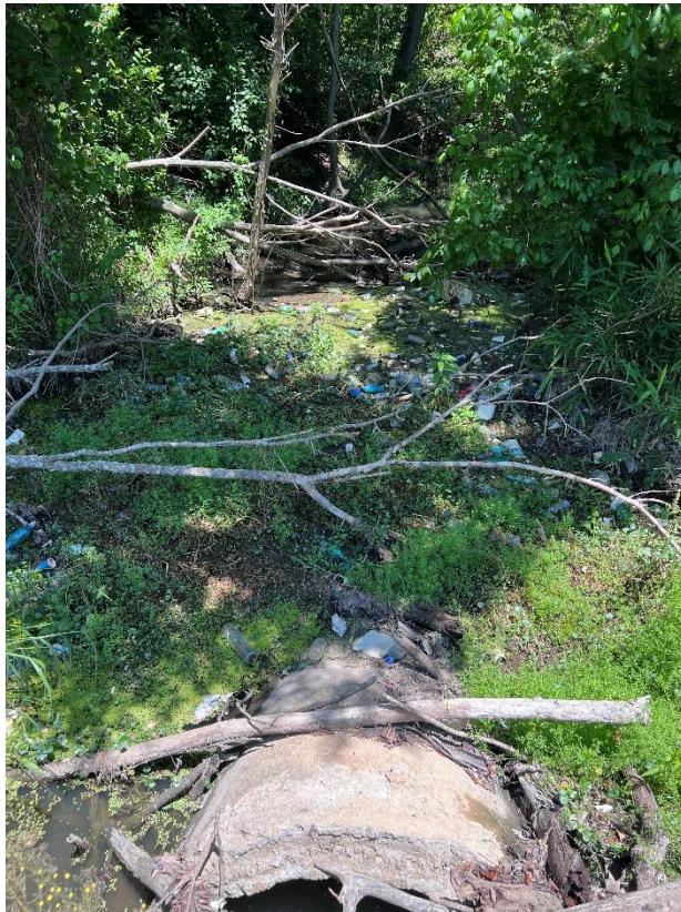
Looking upstream of existing broken 48in RCP
