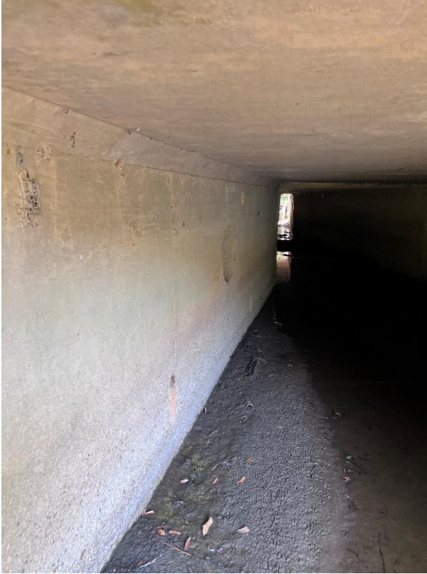
Looking downstream inside 8ft x 6ft RCBC
