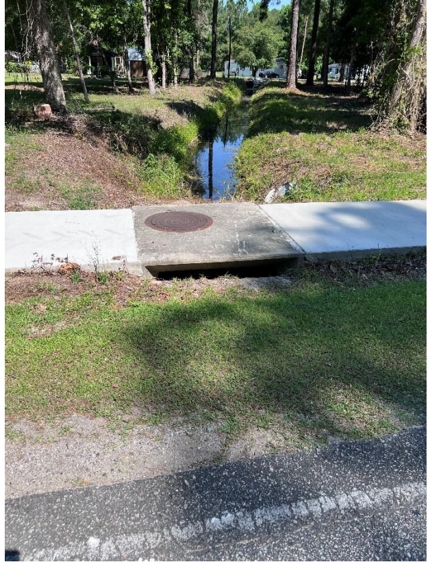
Upstream face of existing 36in CMP
