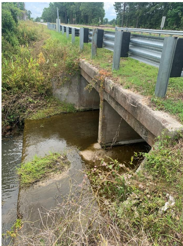
Downstream face of double 8ft x 5ft box culvert
