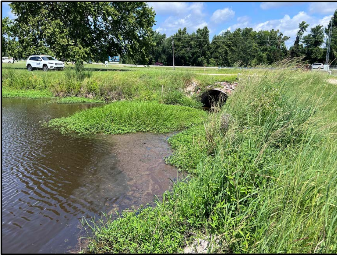
Figure C2: Recent Photo of the 90" x 72" CMP – Upstream Face
