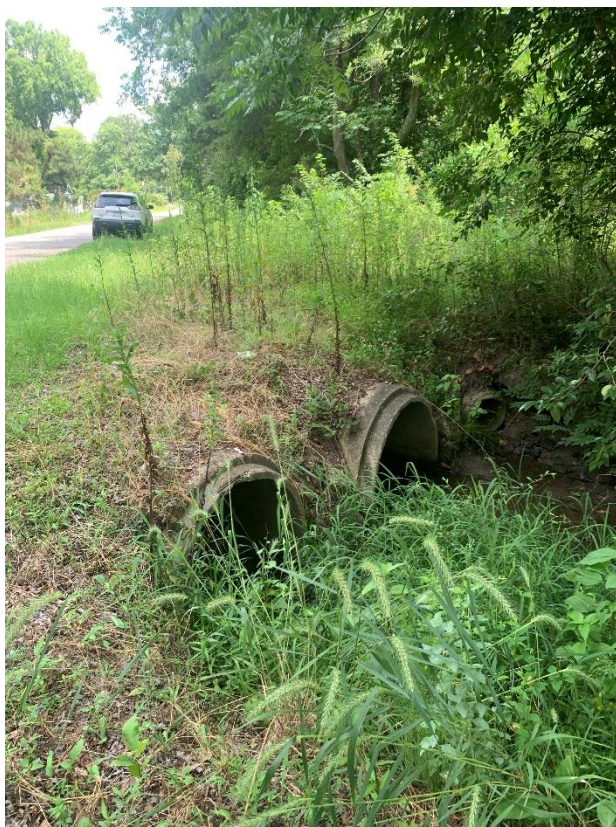
Downstream face of double 48in RCP
