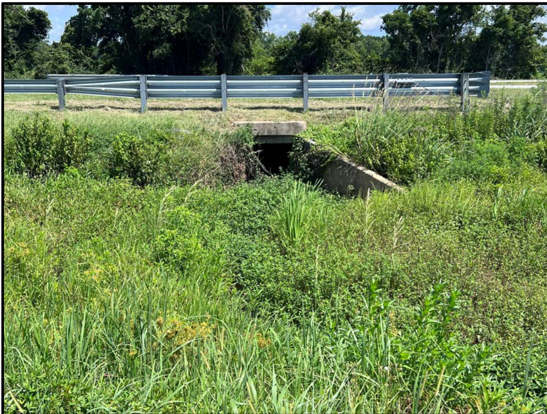
Figure C3: Recent Phot of the 4'(W) x 4'(H) RCBC US 76 Crossing Culvert - Upstream Face
