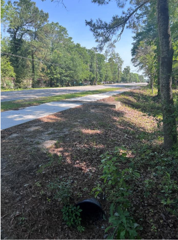
Upstream face of existing 36in CMP
