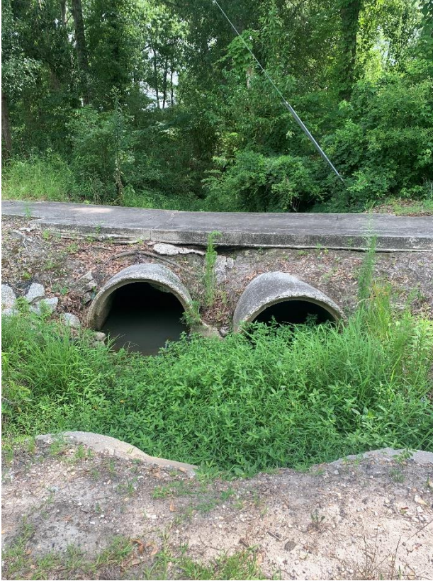
Downstream face of double 48in RCP under sidewalk
