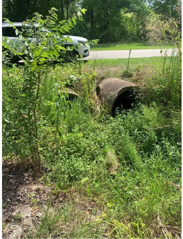
Downstream face of double 48in RCP under sidewalk
