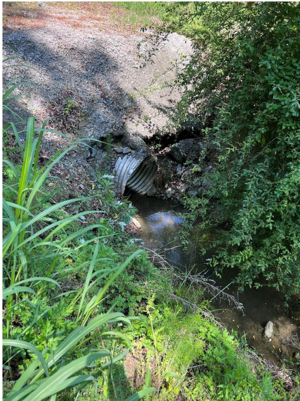
Upstream face of existing 36in CMP
