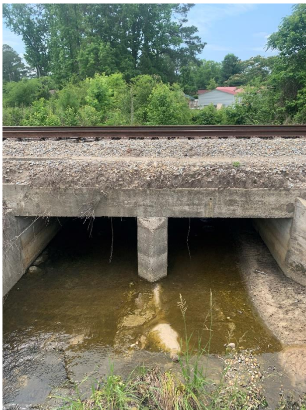
Upstream face of double 8ft x 5ft box culverts under railroad
