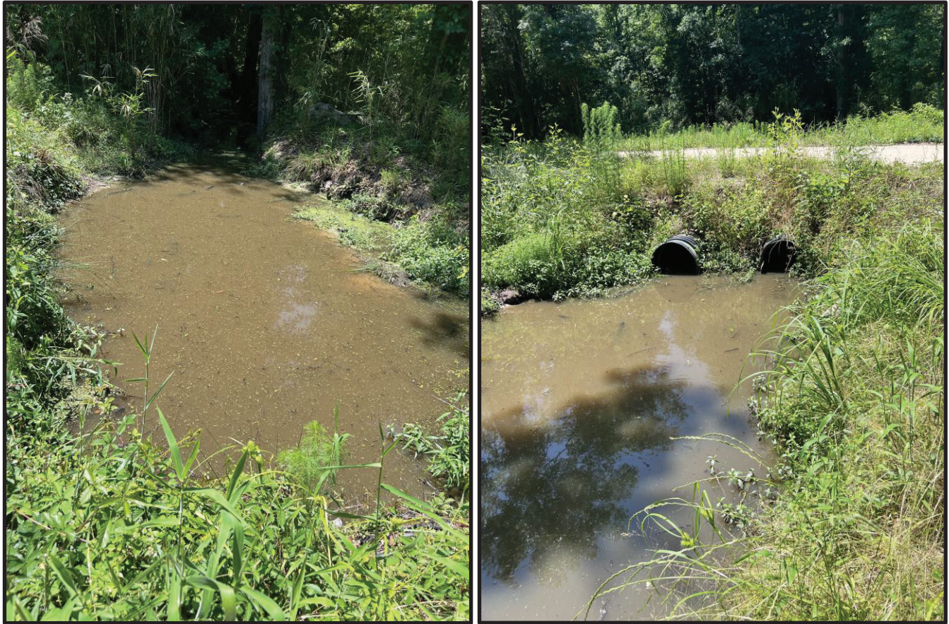
Figures L2 and L3: Awt Road Crossing – Downstream Channel (left), Upstream face of double 24-inch culverts (right)
