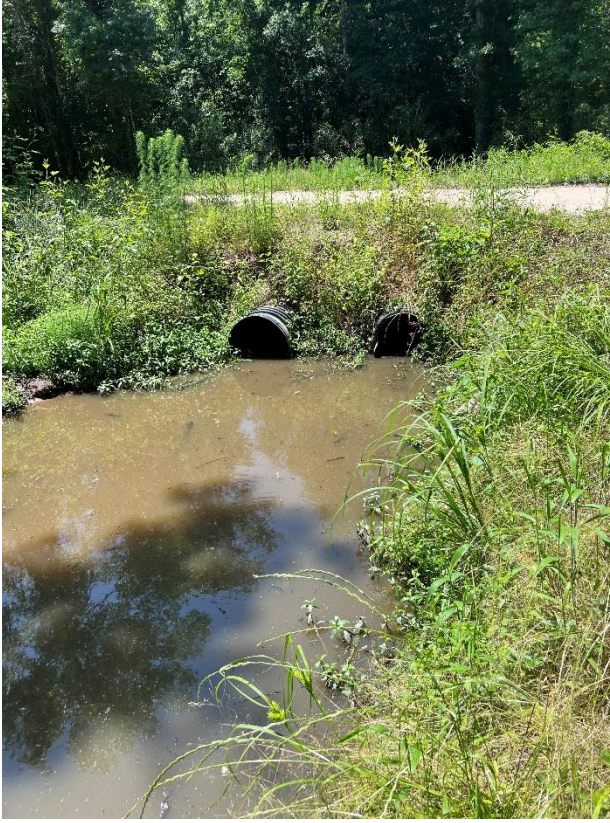
Upstream face of existing (2) 24in HDPE pipes
