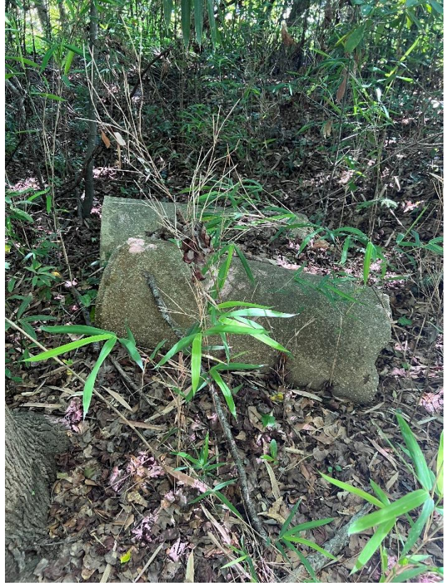
Upstream drop inlet for closed system
