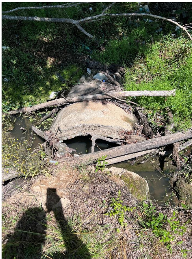
Upstream face of existing broken 48in RCP
