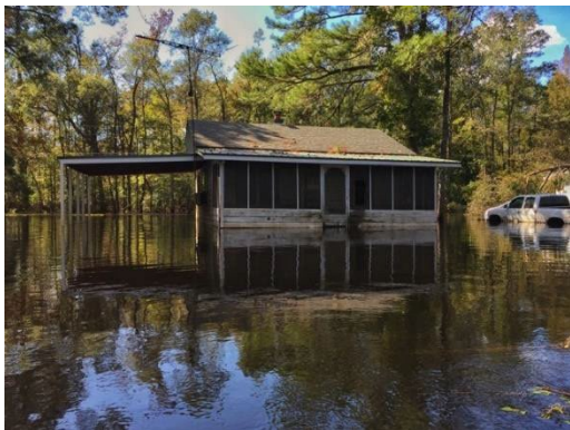
October 18, 2016: Flood waters continued to impact homes in Marion County 10 days after Hurricane Matthew made landfall
