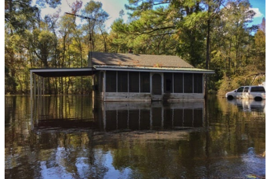
October 18, 2016: Flood waters continued to impact homes in Marion County 10 days after Hurricane Matthew made landfall
