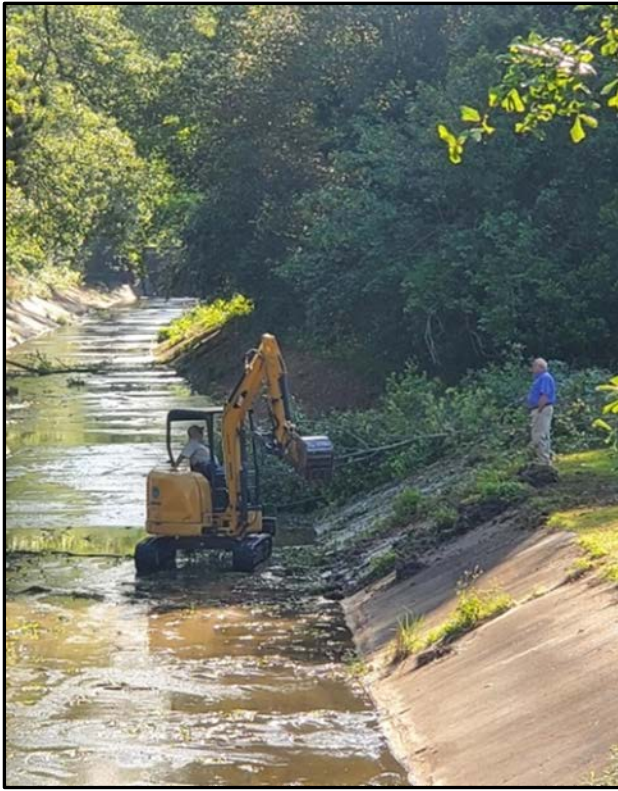
Figure 9. City of Orangeburg Public Works Department cleaning Sunnyside Canal
