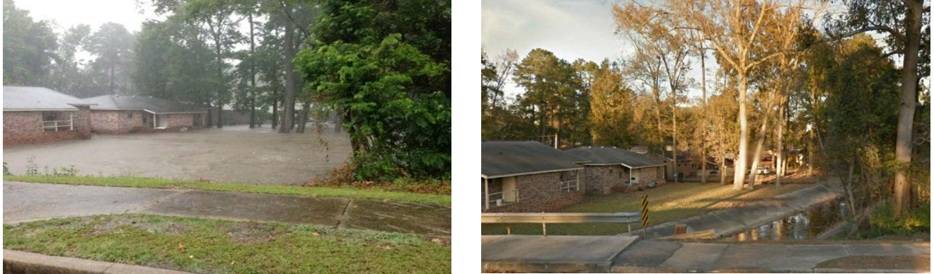
Figure 6. Sunnyside Canal during 2015 flood (left) and during normal conditions (right)
